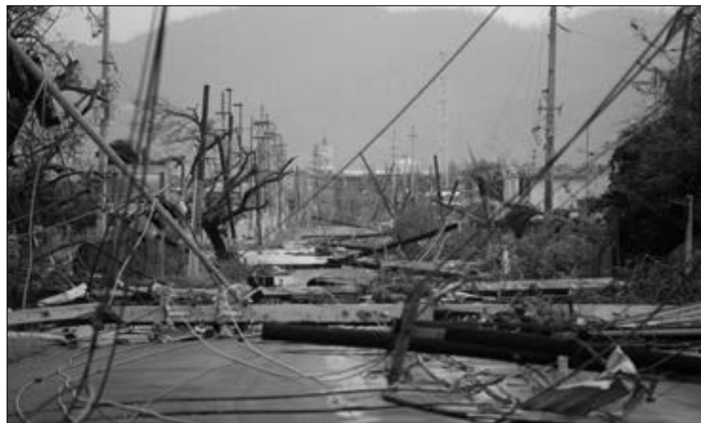
Toppled electricity poles in Puerto Rico following Hurricane Maria
